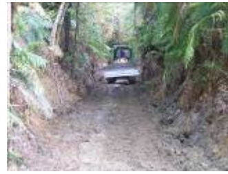
Contractor clearing tramline, credit DOC
